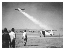
During flight tests on August 21, 1941, the JATO rockets cut the takeoff distance of a small civilian airplane (Ercoupe) by half
